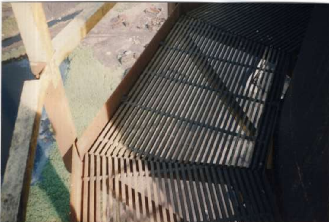
Photo #27 - The grating on the top platform is safe & sound.
