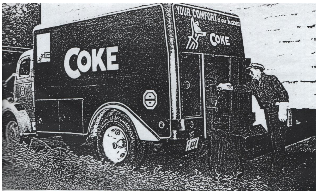
New type conveyor truck for home deliveries of coke.
